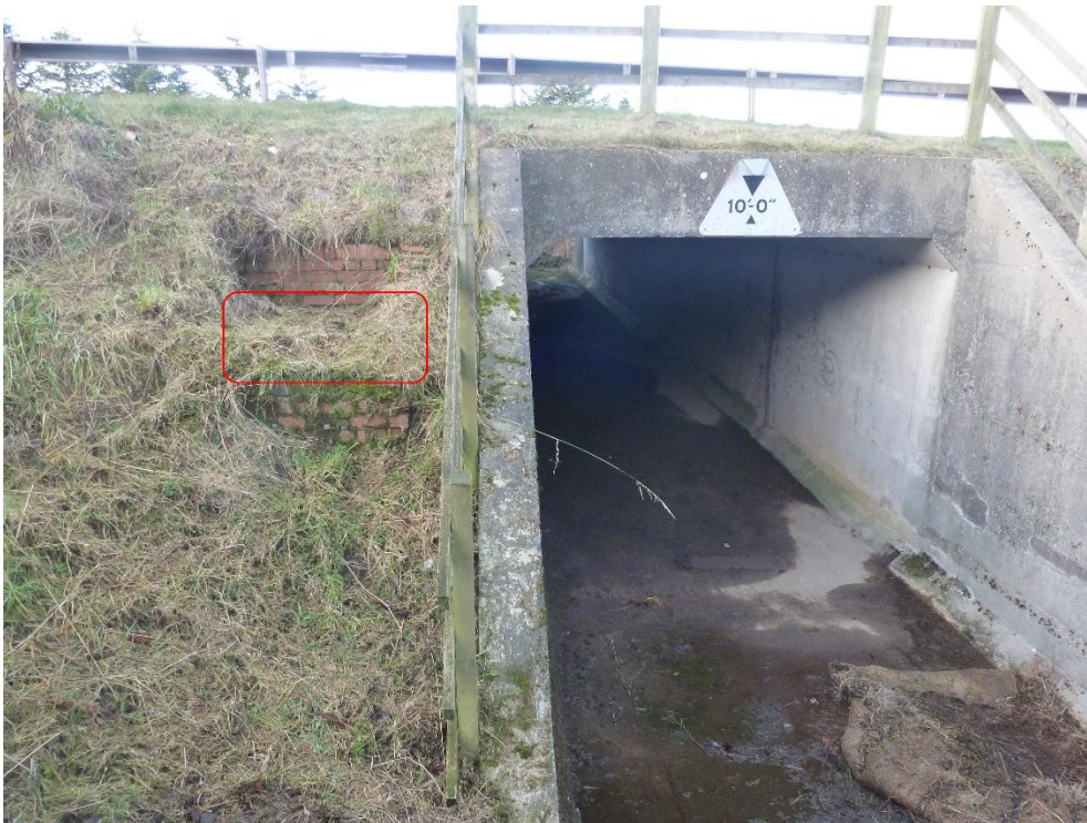
Figure 8 location of manhole cover
