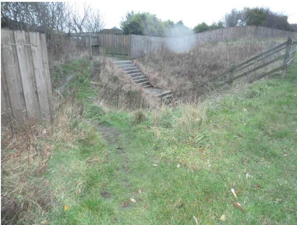
Figure 11 View from A92 towards the underpass steps
