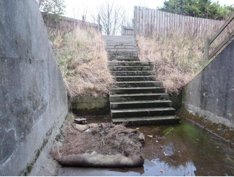
Figure 6 View from the underpass showing the steps from the embankment
