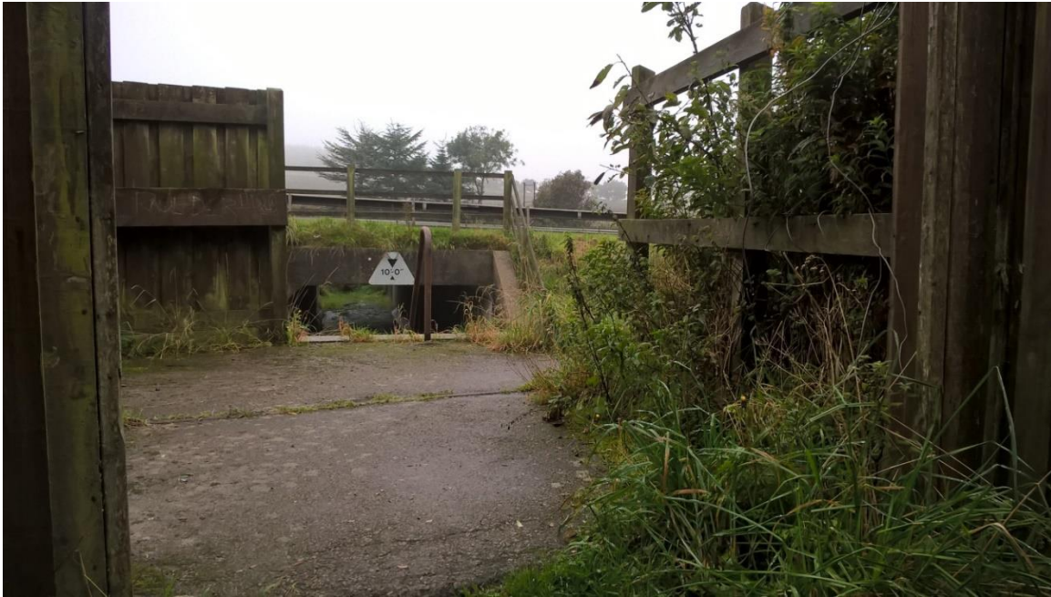
Figure 4 View from the top of the embankment
