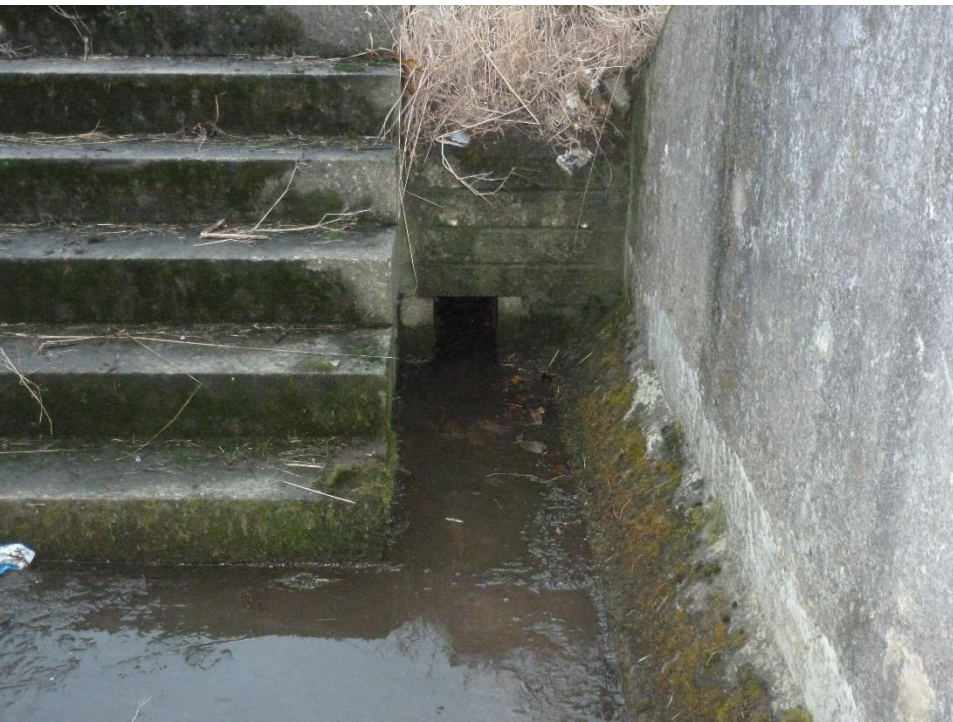
Figure 7 Entrance to drain
